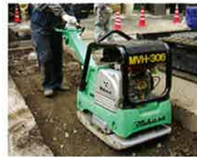
MVH-306DSC 砕石転圧
